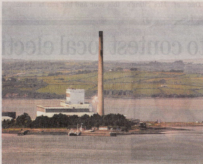
The conversion to gas from coal at Tarbert power station when it is taken over by Spanish giant Endesa will result in half the jobs at the plant being saved, after a complete closure was announced in 2006
